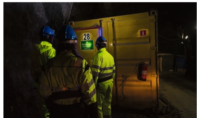
Our Mobilaris Onboard solution works just like your car navigator but without any need for a dedicated tracking infrastructure. In case of emergency, the system helps you to navigate to the closest rescue chamber.
