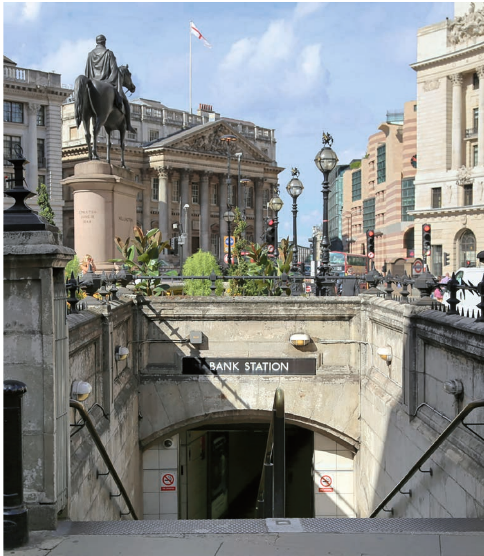
The mining and construction industries serve an important purpose. They have been building communities for centuries – and still do. In London, the construction company Dragados used an Epiroc tunneling ventilation system when they reconstructed the Bank station.
